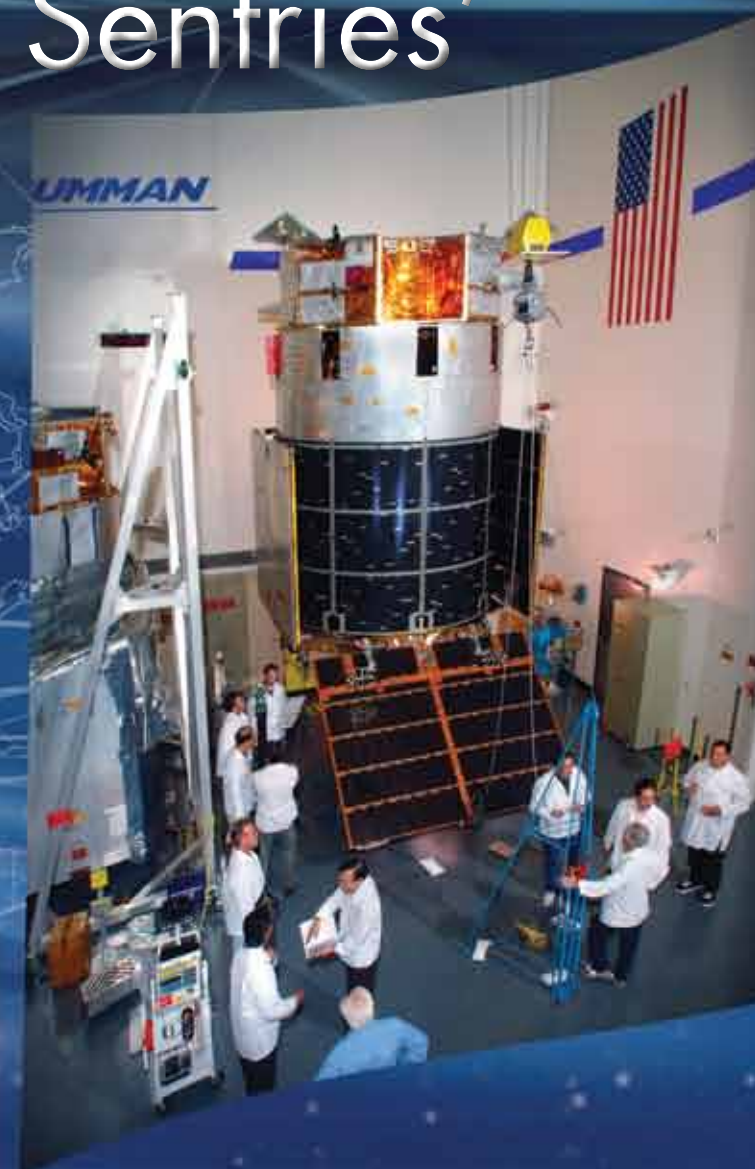
Solar array panels are integrated into DSP spacecraft at Space Park in Redondo Beach, Calif.
